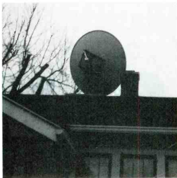
Satellite-TV dish antennas, such as the KLM unit at left, can be ground-mounted affixed to a heavy concrete slab, or as done with the Satellite Receiver Systems' unit, shown at right, roof-mounted. The roof-top installation, which is becoming a common sight in many communities, must be rigidly secured to a sturdy platform to guard against wind-loading, which could turn an improperly mounted dish into a huge airborne saucer.
